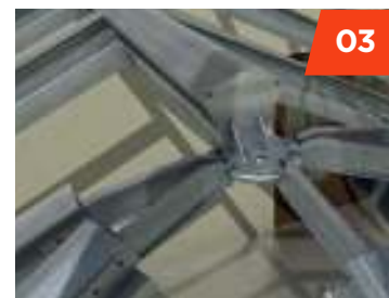
The aluminium rafters, ridges and wall plates are fitted and the spider arms are secured to the spider bracket.
