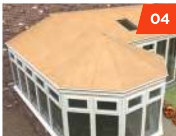
Exterior grade ply-board is fixed to the rafters.
